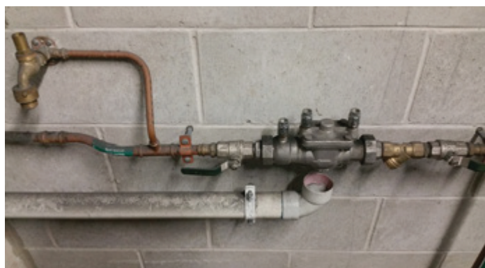
HIGH HAZARD DEVICE IN A BASEMENT
