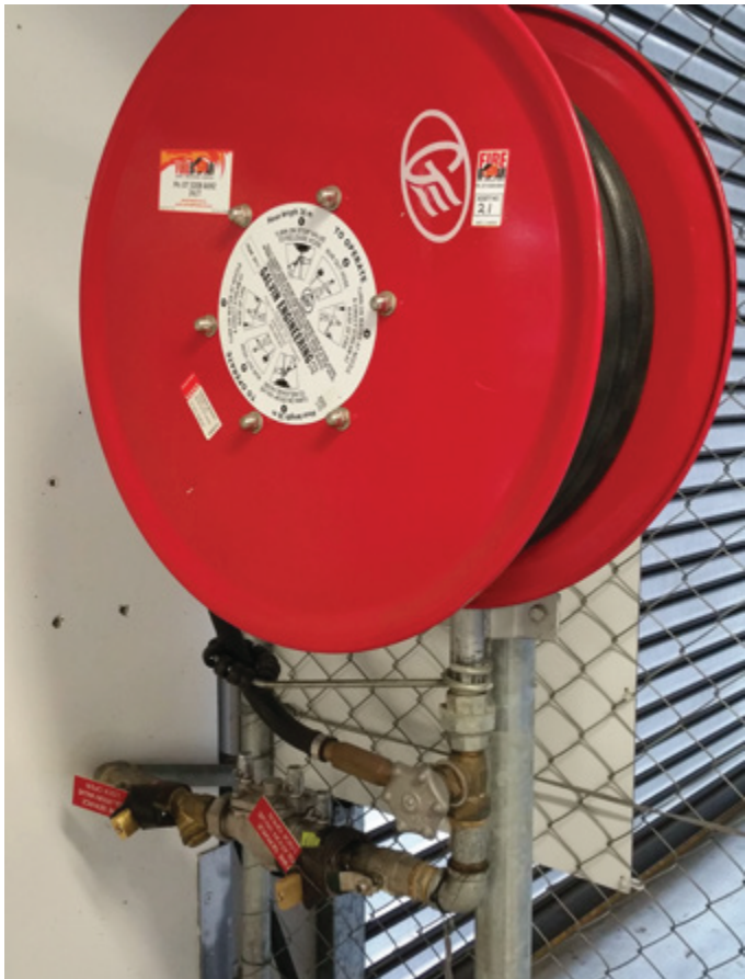
MEDIUM HAZARD DEVICE FOR A FIRE HOSE REEL
