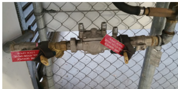
LOW HAZARD DEVICE ON A FIRE SERVICE
